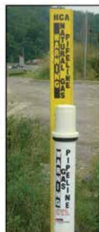
5. HCA marker and cathodic protection test station
