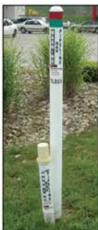
2. Linemarker and cathodic protection test station
