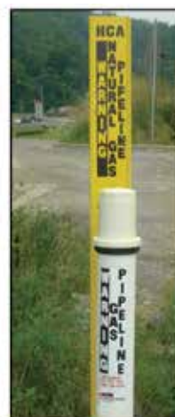
5. HCA marker and cathodic protection test station
